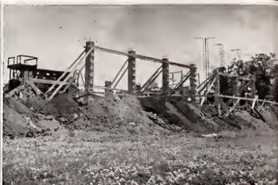
STADIUM GROWS—The new stone and concrete grandstand now under construction at Hardee Field is planned for completion by the end of the summer. The structure, which replaces the old wooden stands, will incorporate a modern press box and other facilities, as well as increasing the possible number of spectators.
