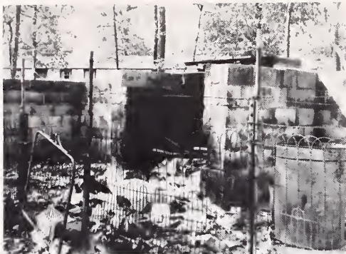
The condition of the incinerator at Woodland has deteriorated greatly in the past year. There is no longer a chimney, nor an effective gate to keep dogs, children, etc. away from the fire and trash. No wonder so many residents are hesitant to light a fire in it.
