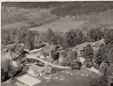
ST. MARY'S FROM THE AIR—Buildings shown in this aerial view of the campus of St. Mary's School are from left to right, the gymnasium, classroom building, main building, chapel. In the background is the riding ring and Cowan valley.
