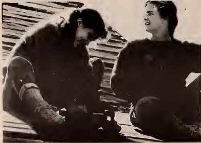
CYNTHIA ELLEDGE and Meredith Stoeber push in to help roof a house in the community as part of Community Building Community (photo by Lyn Hutchinson).
