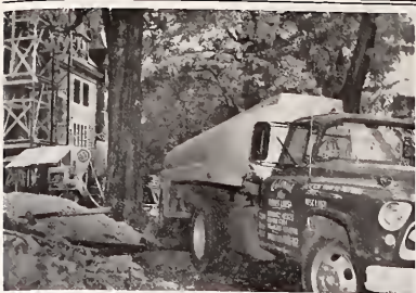
DESTRUCTION AT SEWANEE —During the past week, Sewanee students saw (left) a replacement brought in for the tank truck, being used to supply water for St. Luke's construction, which was pulled off its carriage, punctured, and drained of its precious water supply during the second week of water shortage; and (right) beautiful time-honored landmarks on the corner by the Chapel and Supply Store being leveled to the ground as $1,500 was spent to make parking space for 23 cars.
