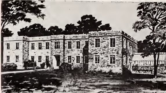
New Snowden Memorial Forestry Building to be ready for occupancy by mid-October nears completion on site next to old forestry building and KS House.
