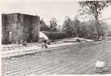
CONSTRUCTION ON JUHAN GYMNASIUM NEARING COMPLETION.—(Left) Floor for new basketball court, which will be surrounded by a 1500 capacity spectator arena, is in process of getting foundation. (Center) Workmen add natural stone exterior finish to the brick wall on the old part of the existing gymnasium. Juhun Gym will enclose the two old very large structures. (Right) The new indoor swimming pool, built on Olympic standards with four lanes, will also have dressing and shower facilities.
