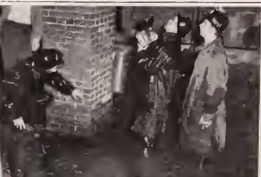
HIVAPY RAINS CAUSE FLOODS ON MOUNTAIN—Members of the Seewanee Volunteer Fire Department aid in pumping water from flooded All Saints' Chapel.
