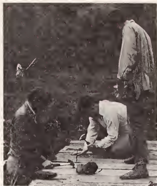
The Sigma Nu's won this year's Help Week project with a renovation of Willie Six Field. The Chi Psi's finished second by reworking the stream behind McCady Hall.
