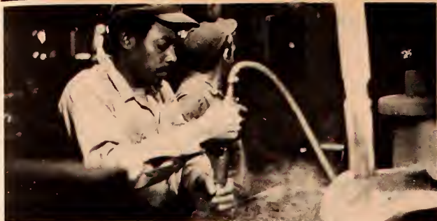
ONE OF THE STEPS IN THE PREPARATION OF SAND MOLDS
