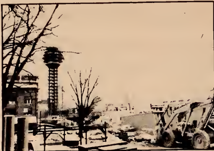
Expo ... Construction on the 1982 World's Fair in Knoxville is still unfinished. (Photo by Jennifer Plant)
